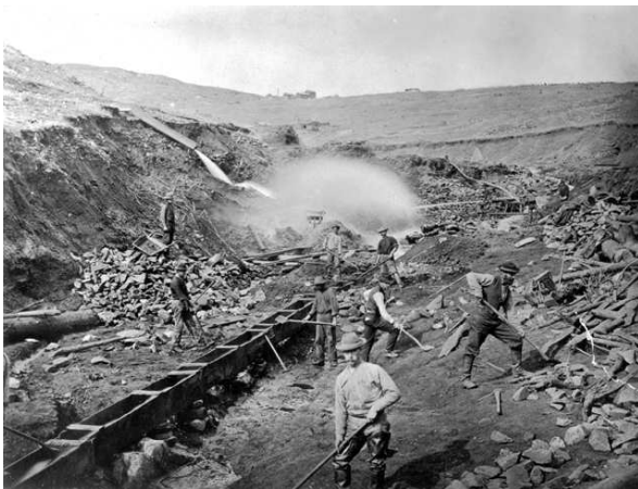
Figure 2-2 Hydraulic Mining in a Clear Creek Tributary during 1877
