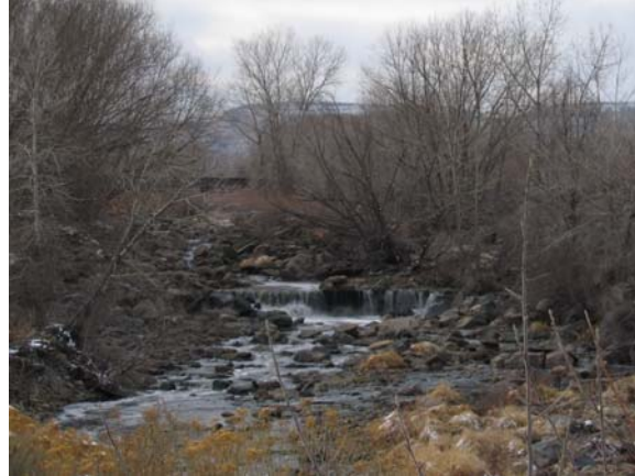
Figure 3-2 Clear Creek Grade Control Structure
